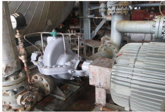
Gambar 1. Pompa Jetting Water
